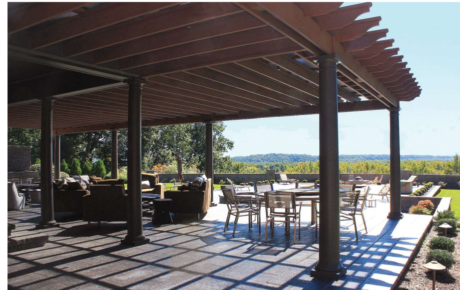
Outdoor living at its finest is achieved with this magnificent pergola. The pergola incorporates a removable ultraviolet screen as the upper layer for sun protection in this southern exposure. While 10% to 20% of the sunlight filters through, the covered area is significantly cooler because hot air is allowed to dissipate through the shade screen mesh fabric. Columns and cedar components are stained a dark brown to complement the home.
