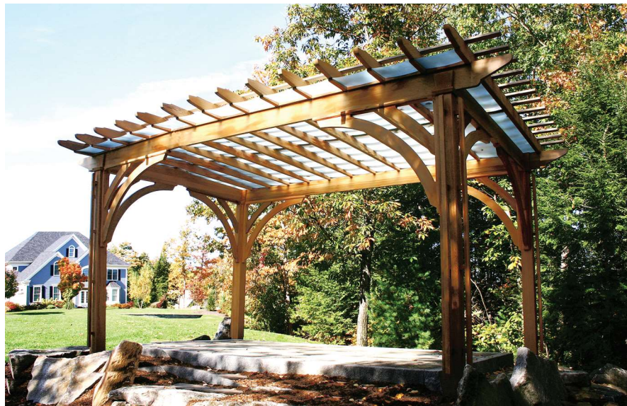
Asked to create an outdoor pergola that would protect the client from rain and sun, we devised a system to incorporate attractive acrylic inserts. These panels are a very soft color with a subtle pattern. Pressed into grooves between the rafters, at a slight angle for drainage, there are no seams and no leaks. Peaked purlins above contribute to additional shade and allow for the growth of vines over the acrylic panels.
