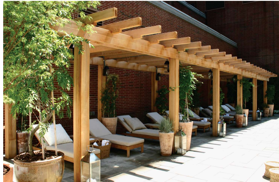
A simple, yet elegant design creates a sun-protected area for lounging at the Soho Grand Hotel in Manhattan. Large boxed posts were created to accommodate a special base attachment we designed for the required codes. Since this structure was to be freestanding, the stainless steel bases had to provide significant lateral support given the contemporary design criteria.
