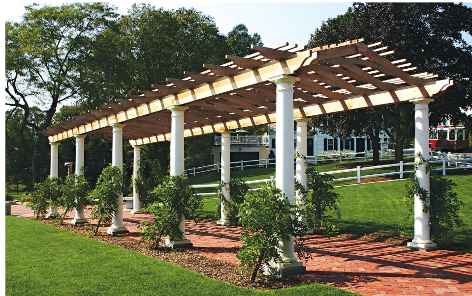
Overlooking the harbor in Plymouth, Massachusetts, this structure was designed to accommodate wisteria plants and to withstand the nor'easter winter storms. In response to this need, we created a special attachment mechanism that also meets the stringent Florida wind load requirements for hurricanes.
