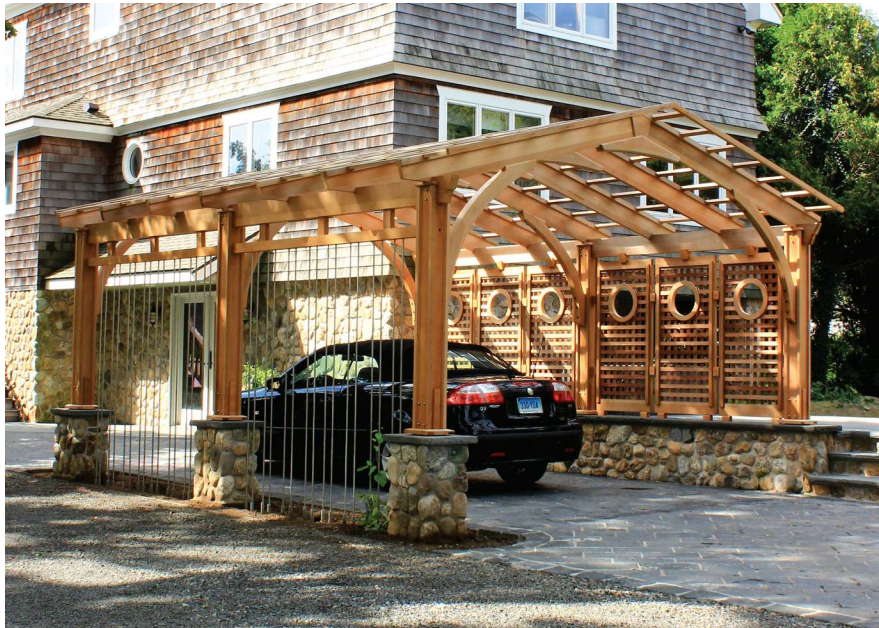
Design elements of the house were incorporated into this carport pergola, such as the large curved brackets, arches and circles within the lattice panels. A contemporary trellis was fabricated using 1/2" stainless steel rods to facilitate a number of vines that within three years time will establish a solid "green screen" in the summer and a intriguing labyrinth of vines during the winter.
