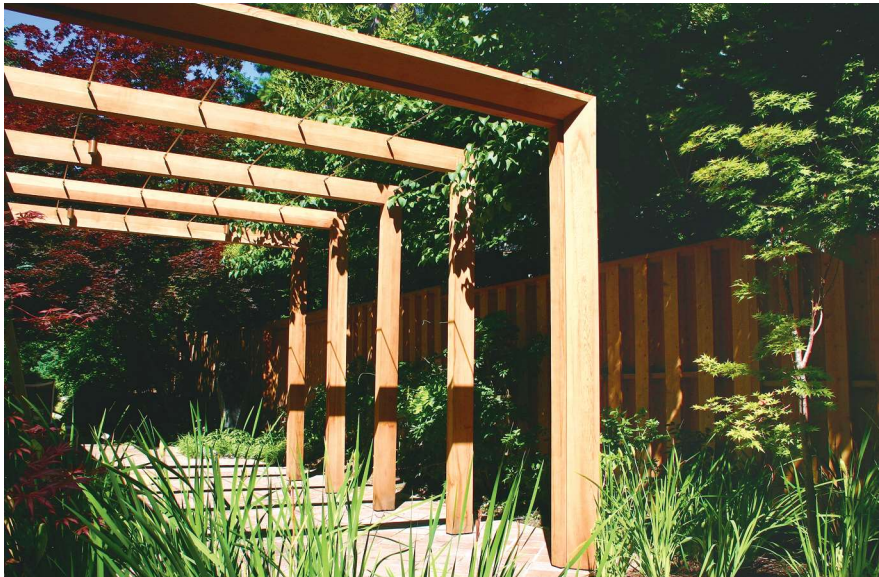
This very simple contemporary pergola incorporates 3/8" stainless rods and stout 6 x 6 posts and beams. The stainless rods were machined to create a very clean, unobtrusive connection to the large beams.
