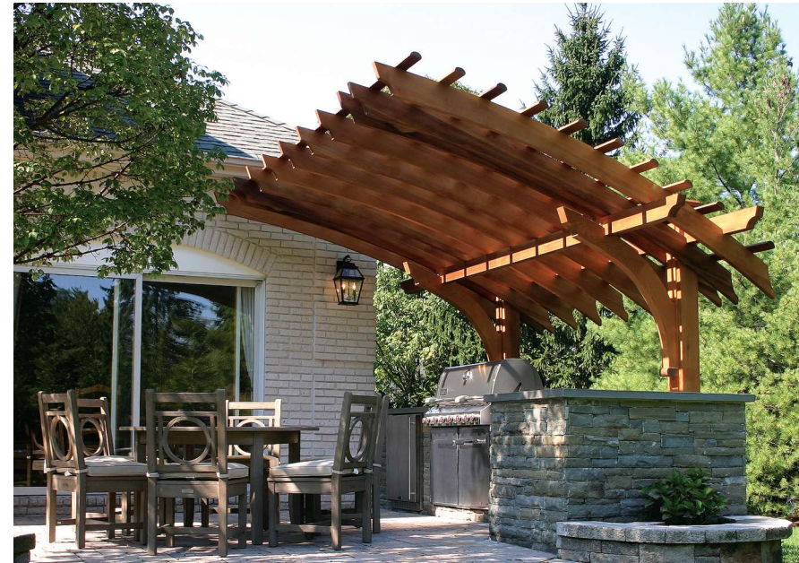
This cantilevered pergola, while maintaining an open feeling, provides a sense of intimacy and privacy in this outdoor kitchen setting. Several unique engineering solutions were incorporated to facilitate the cantilever, thereby keeping the patio free from vertical support posts, per the request of the homeowner. Page 38 of this catalog depicts a few images taken from the 3-D computer model presentation for this project.
