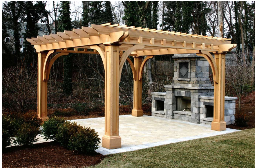
This patio pergola was designed and scaled to go with a large suburban home. The posts are 10” x 10” with plinth bases and large substantial brackets in keeping with the overall proportions. Several architectural details from the house were incorporated in the pergola, creating an open-air extension of the home.
