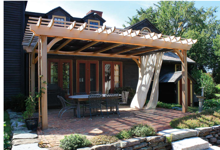
Designed for an early eighteenth century house, this simple pergola has an interesting shade solution. The shade cloth was evenly swagged below the main rafter/purlin layer and is carried by 4 x 4 supports. The upper layers of rafters and purlins are now available as vine support. The vine can co-exist with the shade cloth. Each post has a simple trellis to support the climbing vine.
